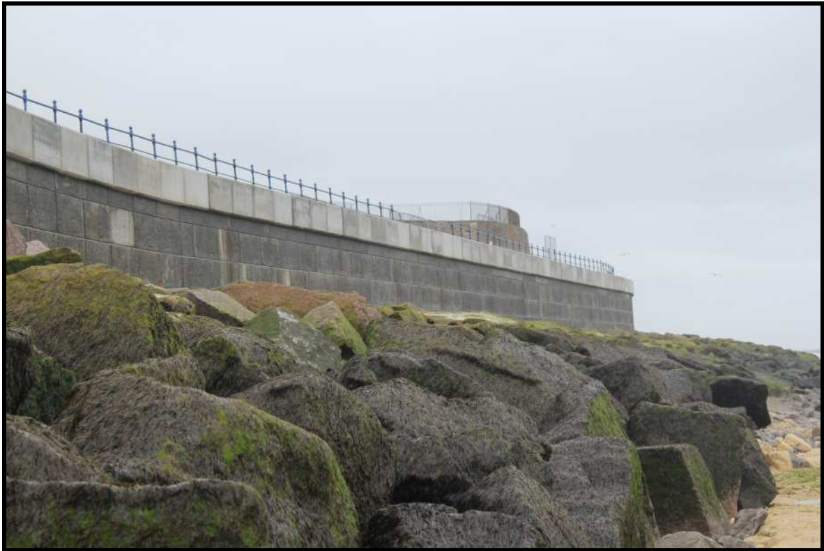
Recent/ongoing construction works viewed looking north from apex of Headland (/C0303C02)
