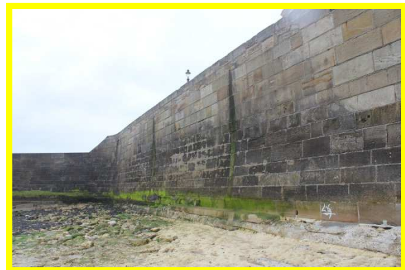
View on masonry wall looking south (/C0303C02)
