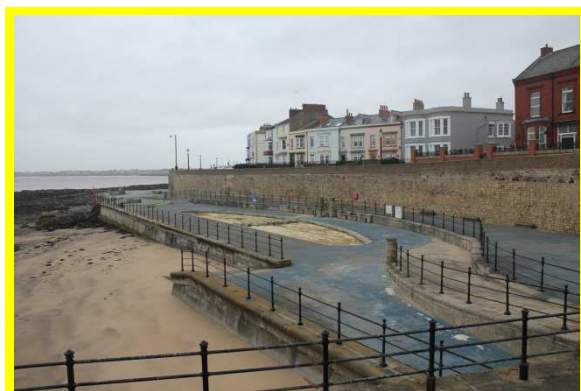
View looking south from Heugh Breakwater (/C0401C04)
