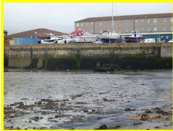
Masonry seawall to north of harbour entrance (/C0401C24)
