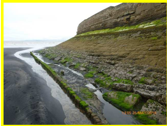
North face of North Pier (/C0401C22)
