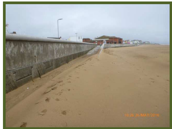
Ridge of wind-blown sand. Note partially buried access ramp (/C0501C03)
