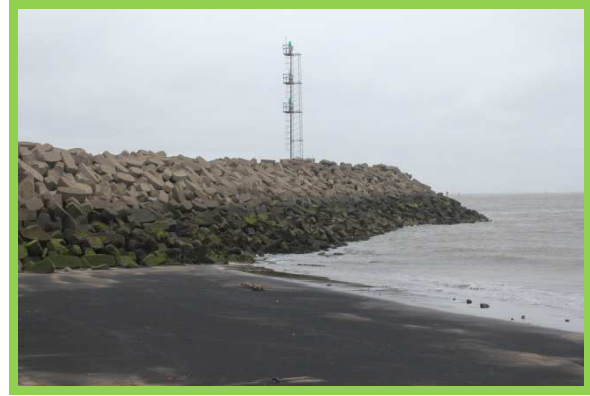
Middleton Jetty south aspect (/C0401C16)
