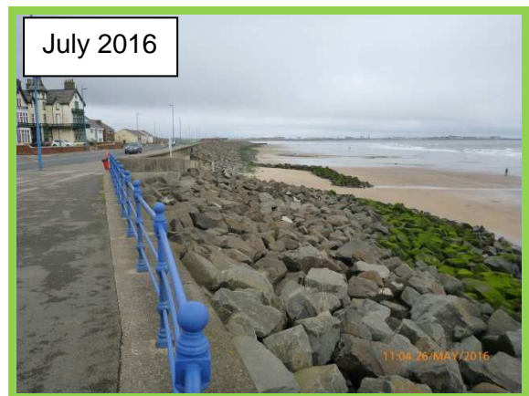
Little Scar access ramp (/C0401C33)
