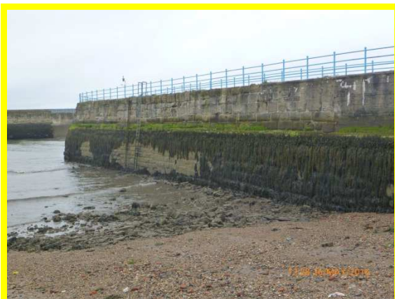
Inner face of Middle Pier (/C0401C28)
