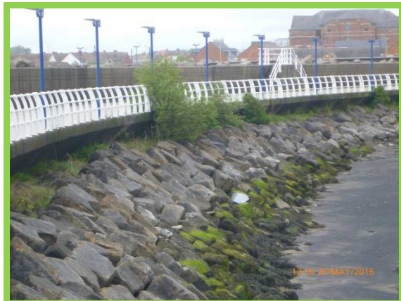
Inner face of South Pier – mature vegetation to be removed (/C0401C32)
