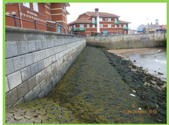
Concrete blockwork revetment obscured by vegetation (/C0401C25)
