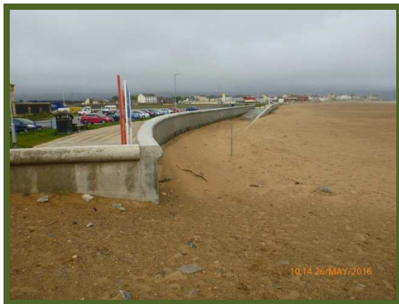
Southern extent of seawall (/C0501C02)
