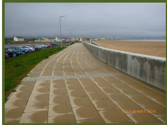
Promenade at pumping station (/C0501C02)
