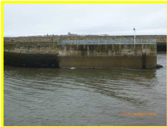
Head of inner arm of North Pier (/C0401C21)
