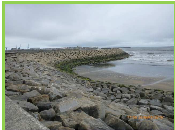
Outer face of South Pier (/C0401C32)
