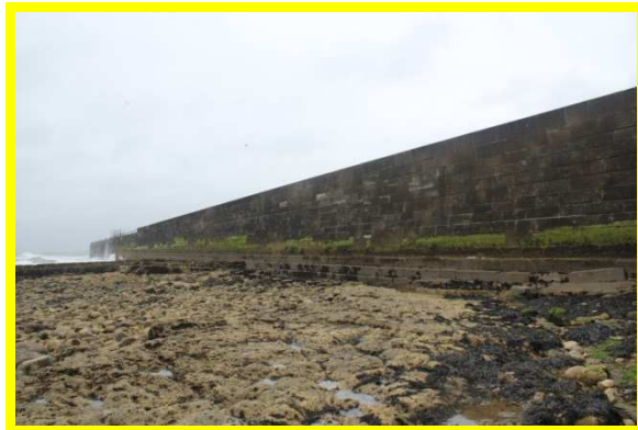
Heugh Breakwater - North aspect (/C0401C01)
