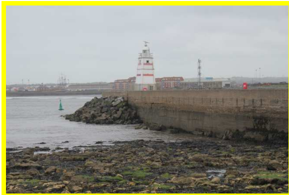
Outer face of North Pier (/C0401C34)
