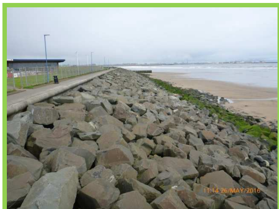
Rock armour revetment and concrete seawall (/C0401C33)
