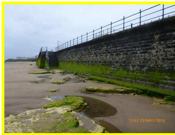
View looking south towards central access steps (/C0303C01)
