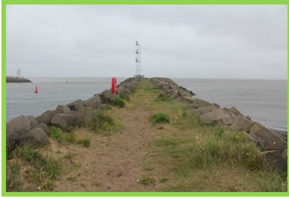
Middleton Jetty north aspect (/C0401C16)
