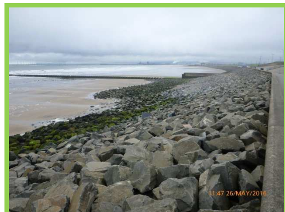
Possible displacement of rock (/C0401C33)
