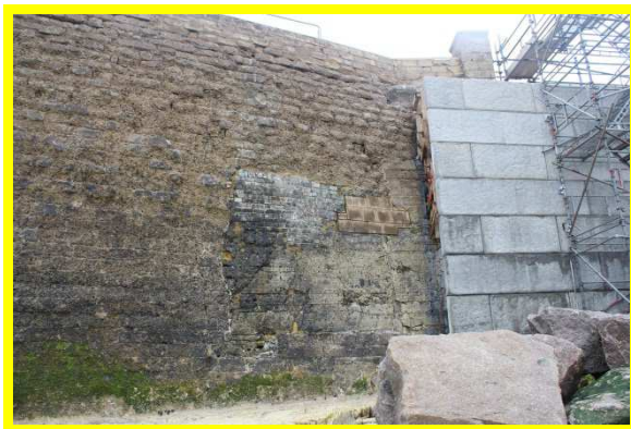
Southern extent of ongoing construction works. (/C0303C02)
