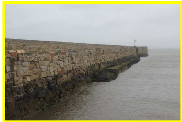
South face of North Pier (/C0401C22)
