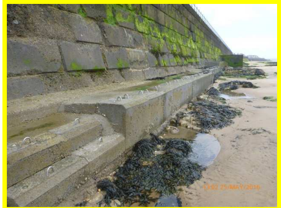
More recent concrete toe protection (/C0303C02)
